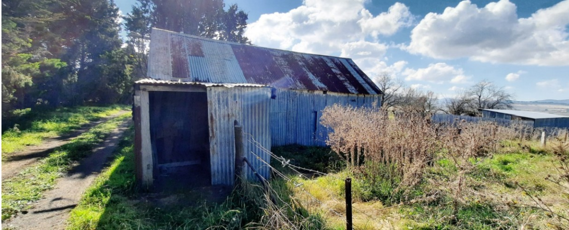
The small (4m x 9m) pole framed shearing shed is a highly intact example of an early vernacular building.
