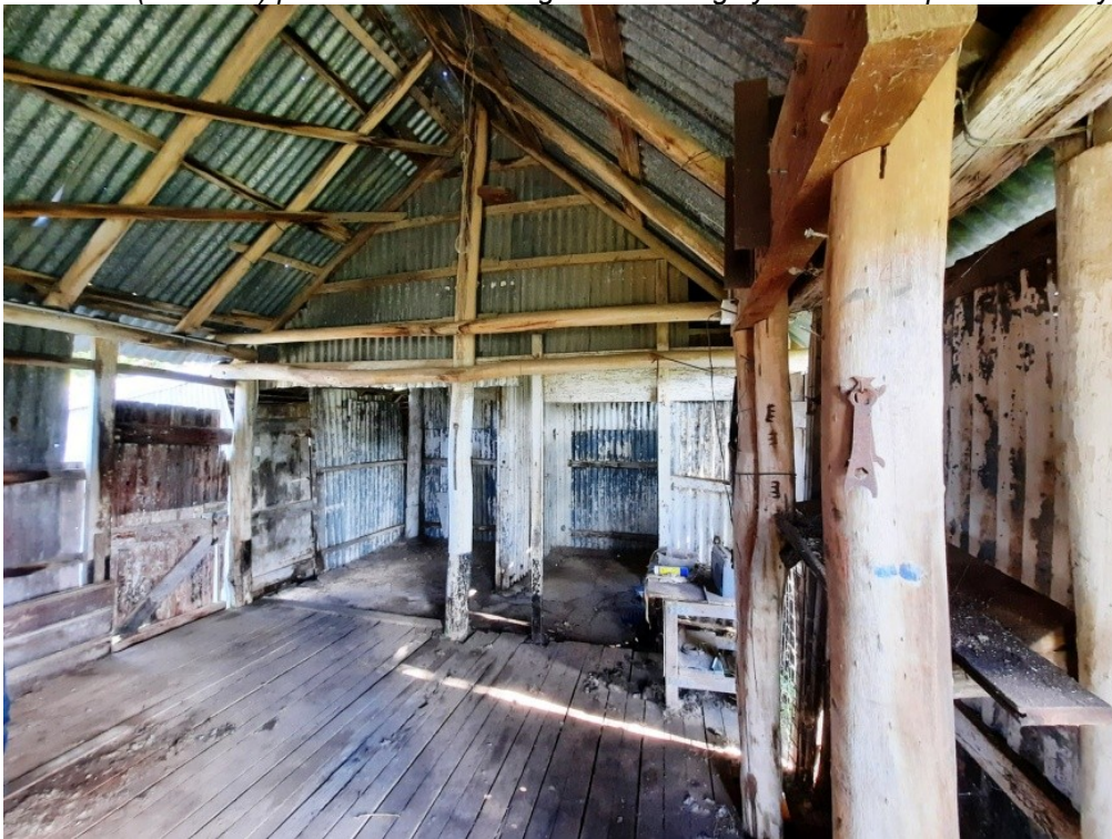
Interior photos showing heritage significant interior details, including roof pole framing, pole posts, slatted floor, galvanised cladding and stalls.
