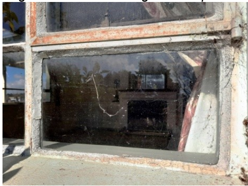
Timber windows were replaced with steel and aluminium framed ones in the 1950s and 1960s.
