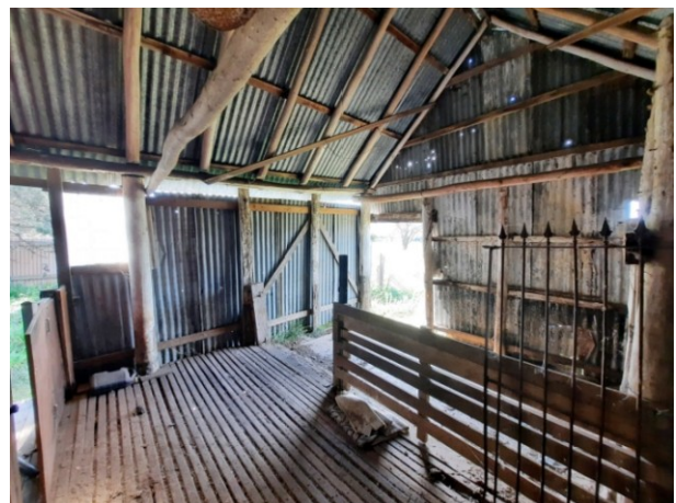
Interior photos showing heritage significant interior details, including roof pole framing, pole posts, slatted floor, galvanised cladding and stalls.
