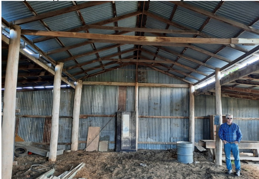
The hay shed main pole frame supports sawn timbers..
