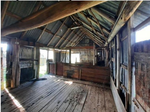
Interior photos showing heritage significant interior details, including roof pole framing, pole posts, slatted floor, galvanised cladding and stalls.
