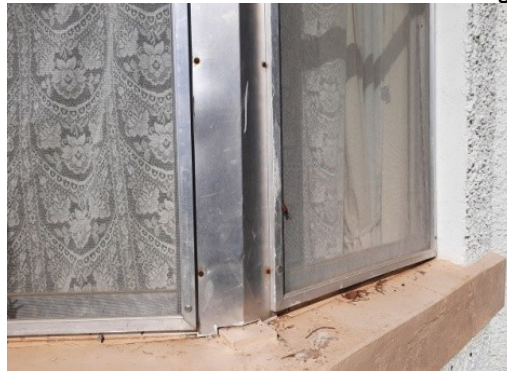
Timber windows were replaced with steel and aluminium framed ones in the 1950s and 1960s.
